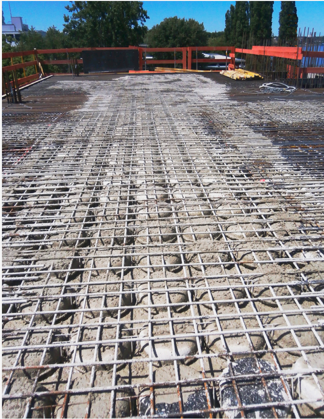
Void former in installed condition / 1st concreting (Source: Fritz Meyer GmbH)
