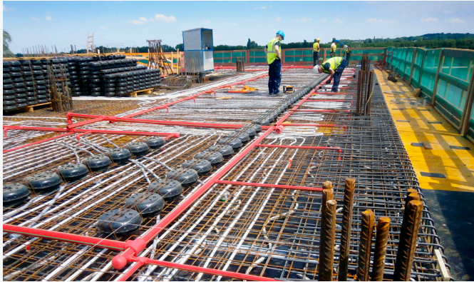
Alignment and securing of the first row of void formers S120-140c (Source: Fritz Meyer GmbH)
