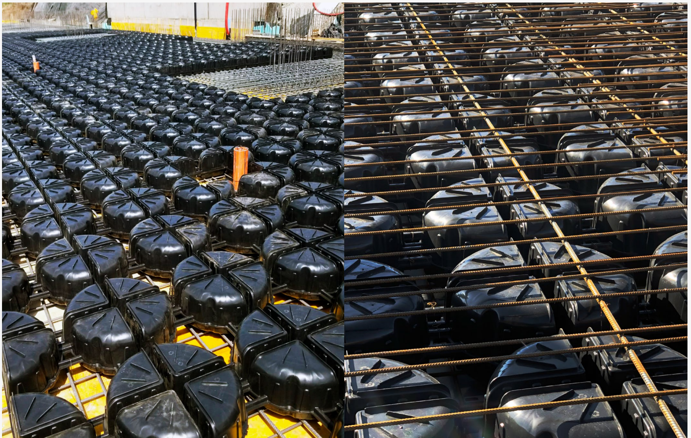
Globally, more than 14 million square metres of Cobiax voided flat slabs have been produced to date. This corresponds to a saving of 2 million tonnes of concrete and a reduction of 180,000 tonnes of CO 2 . Images: © Heinze Cobiax Deutschland GmbH
