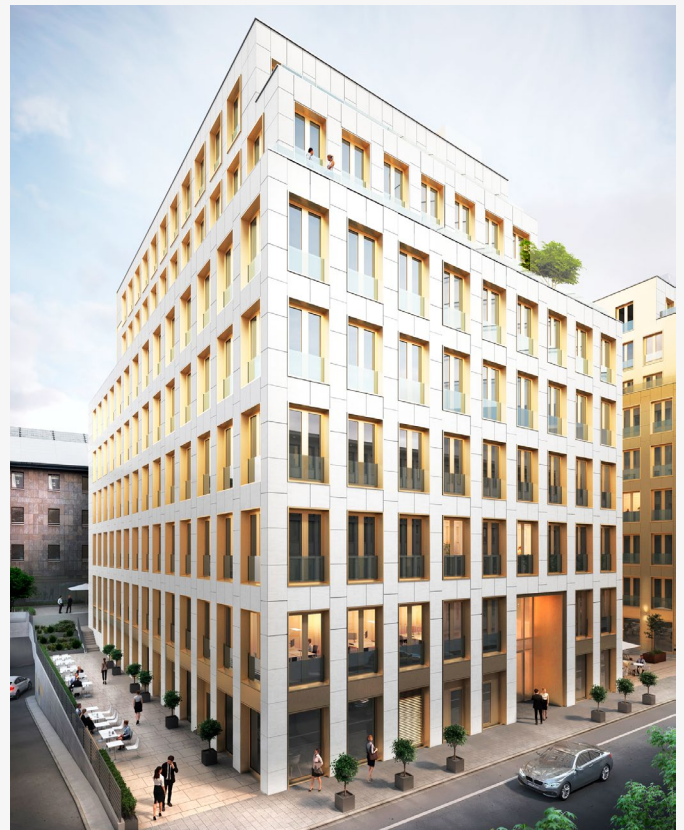
Two-storey galleries and the open and friendly façade design lend the new building an attractive look and an individual personality.
