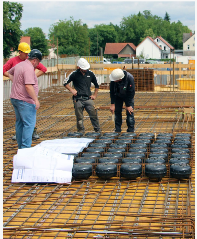
Construction meeting: The installation plan is implemented exactly. Source: Aller-Weser-Klinik gGmbH.
