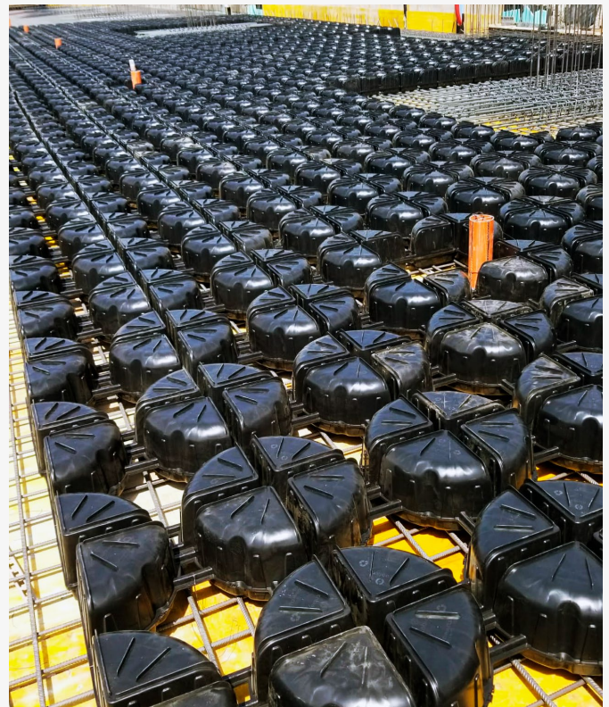
The modules can simply be joined together in rows and so form a solid structure. Source: Heinze Cobiox Deutschland GmbH
