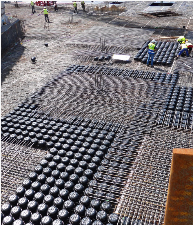
Void former modules from Cobiax are used to keep the weight of the building constant despite its getting taller. Source: CEMAGG Weil am Rhein GmbH & Co. KG
