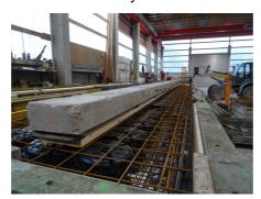
There was no significant difference between the concreting and compressing procedure and the procedure used for the conventional prefabricated slabs. It was performed swiftly. The concrete used was C35/45 of the F4 consistency class.
