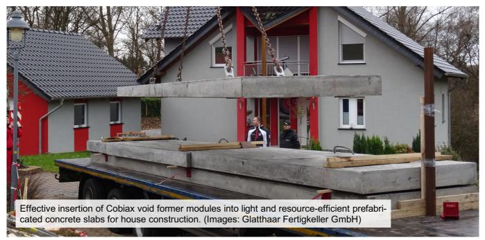
Commissioned by a prefabricated house manufacturer, the companies Glatthaar Fertigkeller GmbH & Co. KG and Heinze Cobiax Deutschland GmbH have successfully studied how to insert the Cobiax void former systems into prefabricated concrete slabs as a practical example for house construction.
