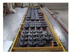
The modules were flexibly shortened and partially connected using a binding wire and secured against dislocation with the reinforcement. The edge reinforcement and the upper reinforcement layer were subsequently installed. The Cobiax void former modules simultaneously serve as a supporting element in this case.
