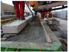
After removing the load, the nonconcreted areas were filled in, re-compacted and the entire surface was smoothed out.
