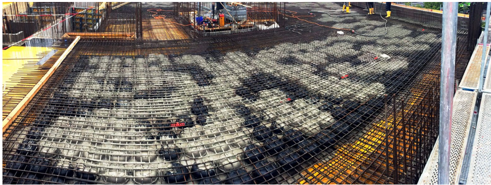
An upcoming Cobiax SL reinforced concrete slab during the first concrete casting process.
