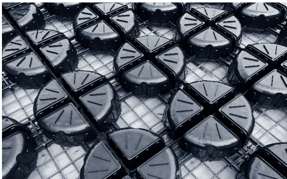
Laying of the void formers close together without gaps acc. to Cobiax installation plan, smaller half-shell at the bottom
